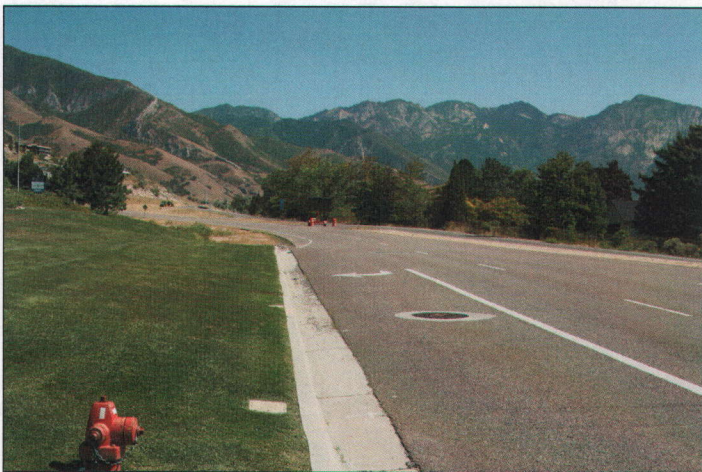
Looking east on Parleys Way from its intersection with Wilshire Drive. Traffic coming from this direction is from either Foothill Drive, I-80 or I-215. A single lane heads in this direction for access to I-80 or I-215.
