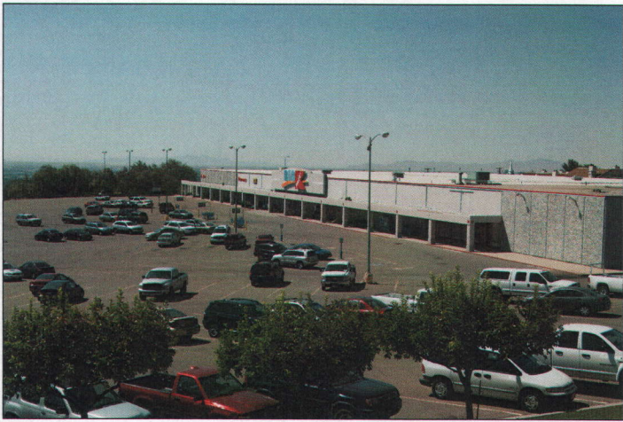
The Kmart building as viewed from the neighboring office building.
